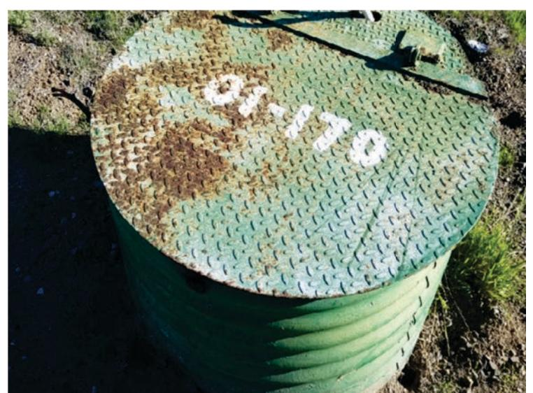
Photograph of an existing monitoring well onsite
